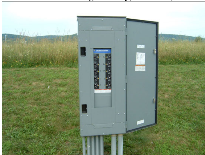
Figure 4. Distribution Panel Receiving 300 amp, 460 VAC, 3-Phase Electrical Feed
