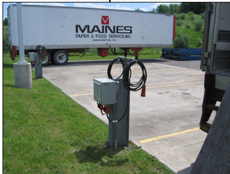
Figure 6. I-Beam Equipped with 460VAC Electric Power Shown with New Wiring and Power Receptacles Installed
