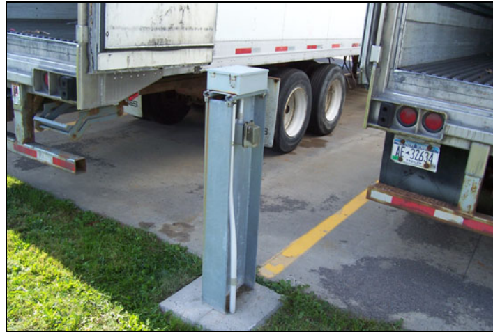
Figure 5. I-Beam Equipped with 110VAC Electric Power Shown Prior to eTRU Connection Installation
