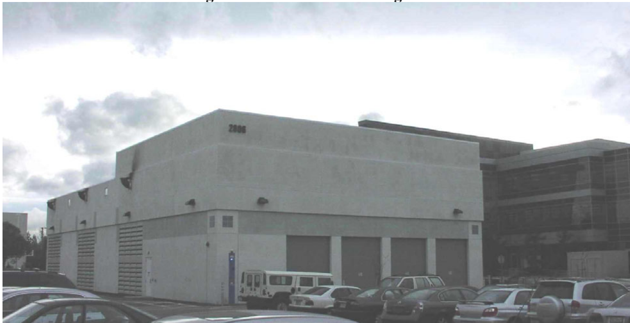
Figure 3. New Central Cooling Plant
