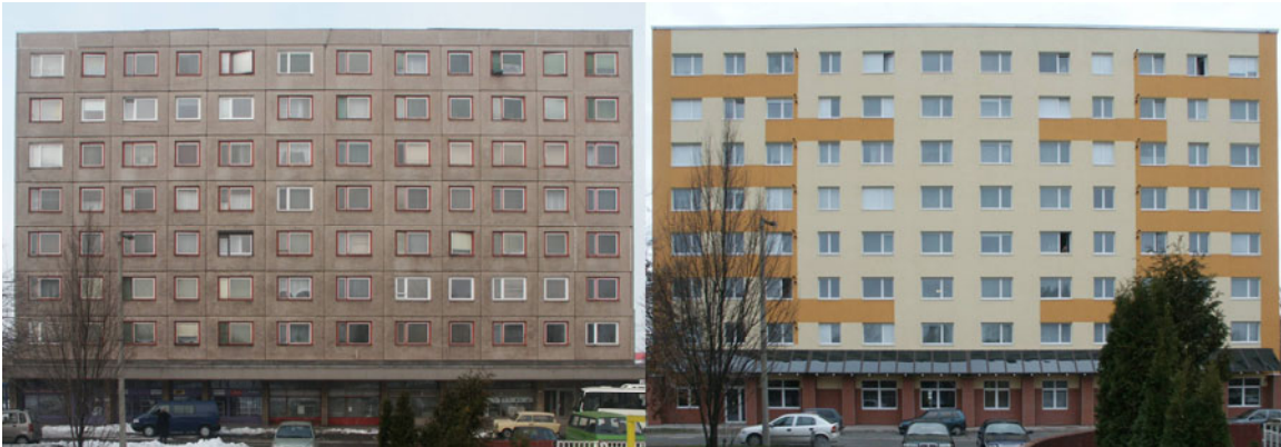
Figure 2. SOLANOVA Demo Building Before and After Retrofit, Southern View
