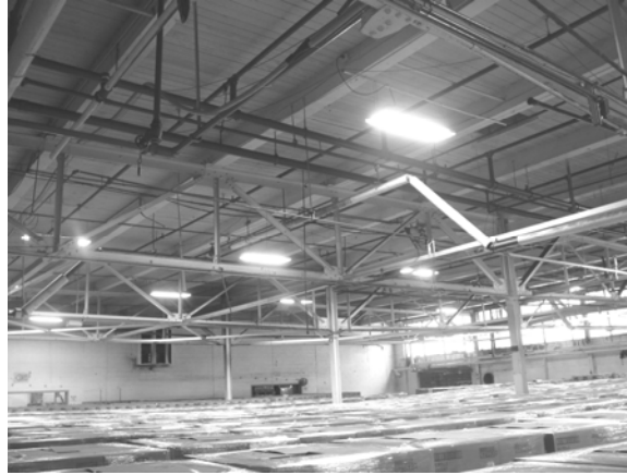
Figure 2. Warehouse Area After Installation of New Lighting System
