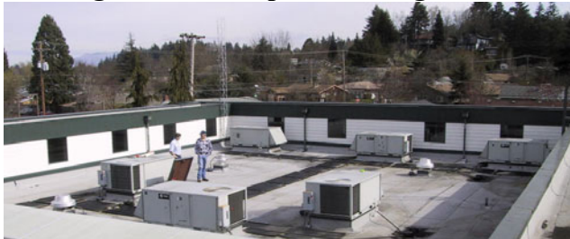
Figure 4. Rooftop of Building “A”
