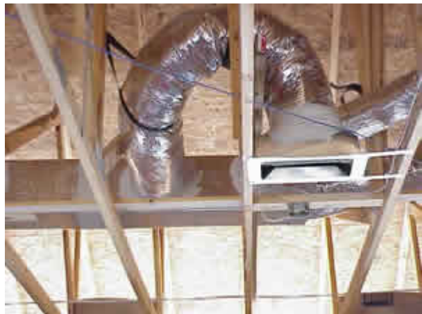
Figure 6. Mastic Sealed Attic Supply Duct and Plenum
