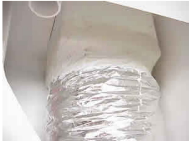
Figure 6. Mastic Sealed Attic Supply Duct and Plenum
