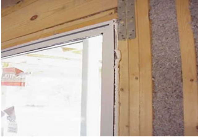
Figure 7. Good Insulation Detail of Blown Cellulose Installation and Foam Insulation Around Window Frame
