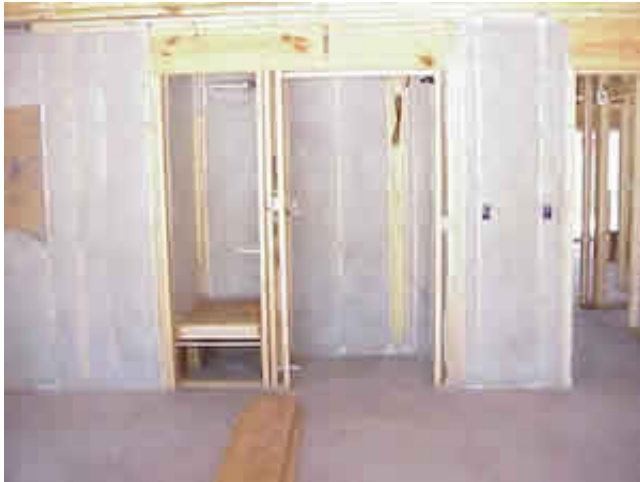
Figure 3. Damp Spray Cellulose Covers Walls of Mechanical Closet (in Condition Space) and Water Heater Cabinet in the Garage. Home Entry is on the Far Right
