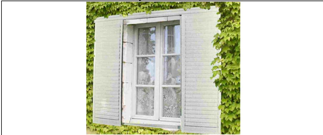
Figure 7. Photo of External Insulating Shutters Made in the US Superimposed Electronically onto a Home in France
