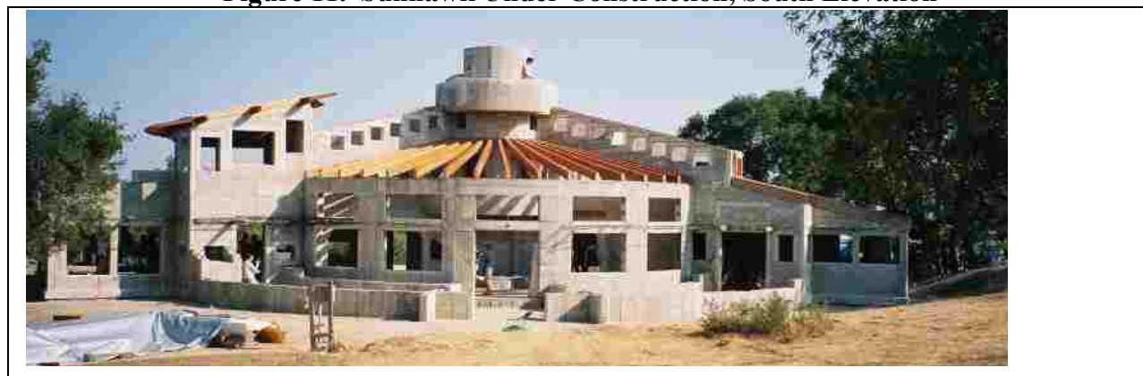
Figure 11. Sunhawk Under Construction, South Elevation
