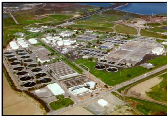
Figure 1: San Jose Water Pollution Control Plant
