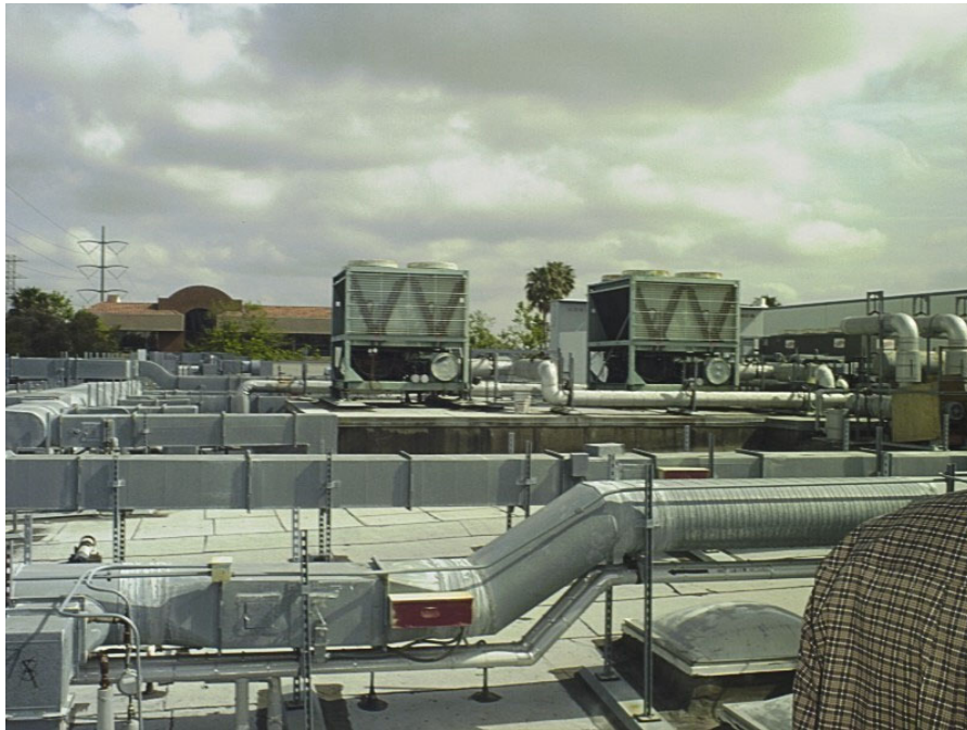
Figure 10. Air Cooled Chillers and Facility Roof
