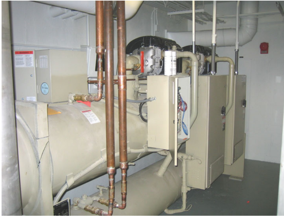
Figure 11. McQuay WMC150 Chiller
