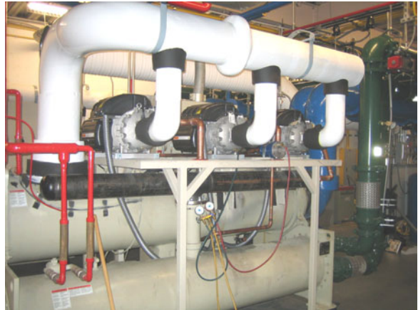
Figure 13. After – 250 Ton Retrofitted Chiller
