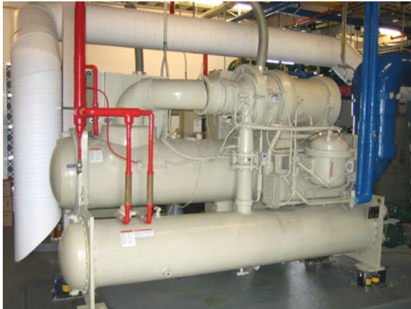
Figure 12. Before – 250 Ton Centrifugal Chiller
