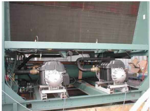
Figure 15. After – 120 Ton Retrofitted Chiller
