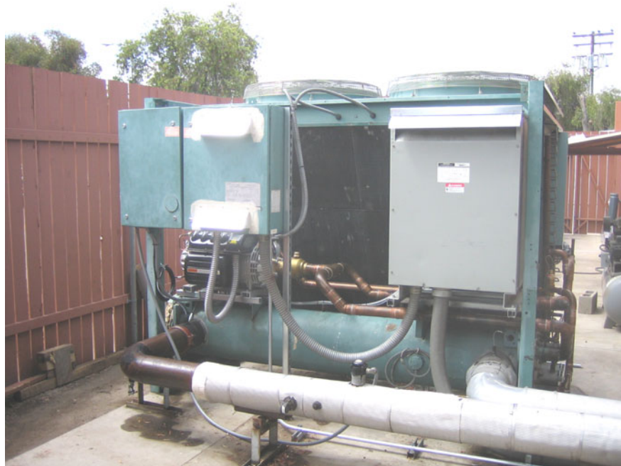
Figure 9. Air Cooled Reciprocating Chiller Post Retrofit
