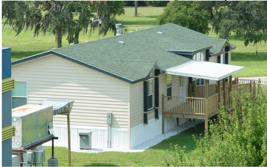
Figure 1. Manufactured Housing Laboratory
