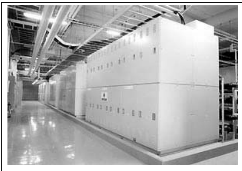
Figure 5. Tottori SANYO Factory VRB Installation
