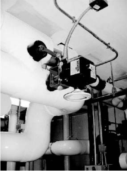
Figure 3. Changeover Valve
