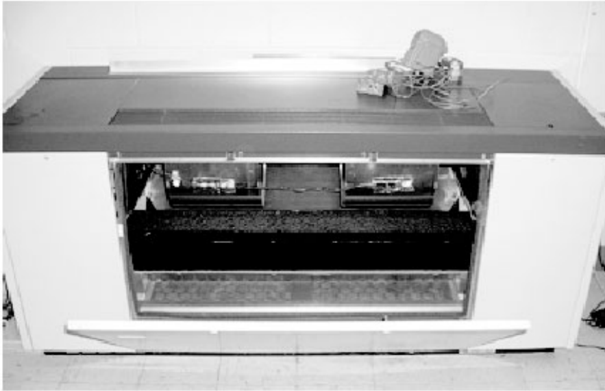
Figure 8. Unit Ventilator with Face and Bypass Controls
