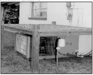
Figure 6. Trellis Shading Device Built over the Condenser at Site #2
