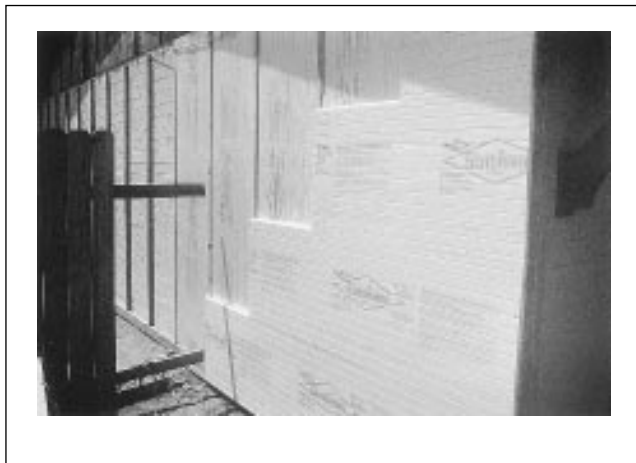
Figure 2. Retrofit Installation on the Arizona Field Test Houses Began by Installing Furring Strips and Extruded Polystyrene Foam Insulation Boards
