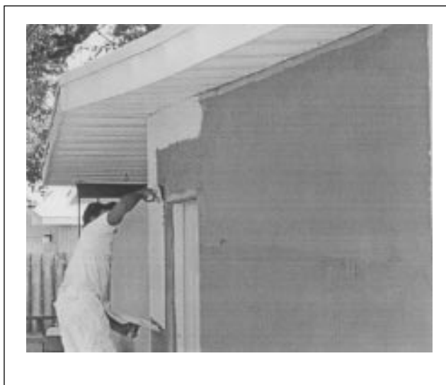
Figure 6. An Acrylic Polymer Finish Mastic Was Applied over the Base Coat of Mastic on the Florida Field Test Houses
