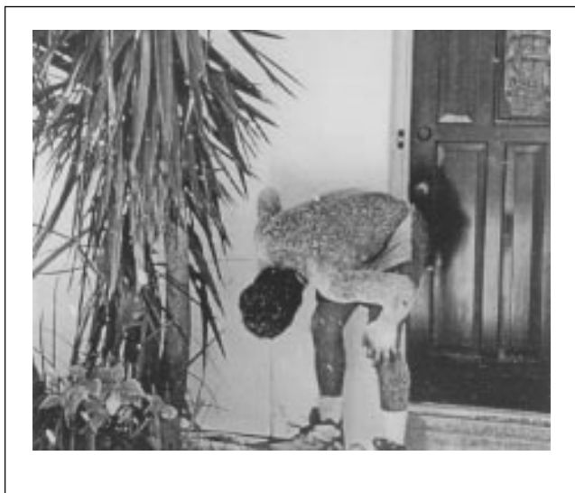
Figure 5. The Extruded Polystyrene Foam Insulation Boards Were Sanded and Planed on the Florida Field Test Houses to Obtain a Smooth Surface
