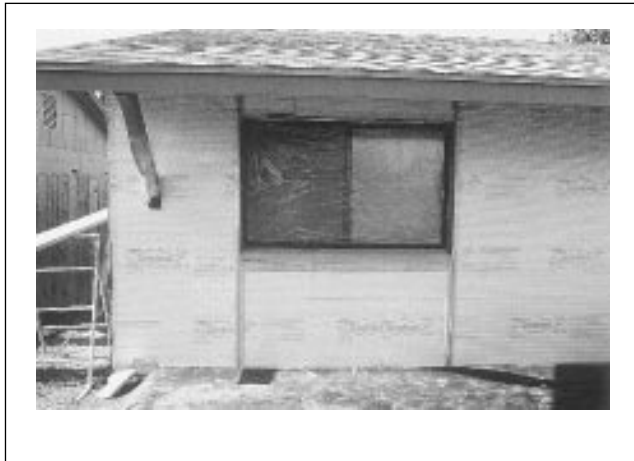
Figure 3. A Wire Lath with Flashing, Metal Trim, and Control Joints Was Installed on the Arizona Field Test Houses Before Applying the Stucco Finish
