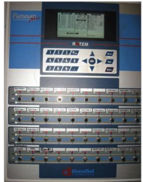
Control panel for poultry house lighting, Oneonta, AL.
