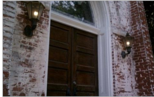
Church with compact fluorescent lighting
