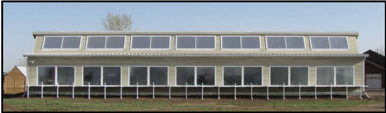
Figure 12. South Elevation of 3000 ft 2 Greenhouse, April 2012
