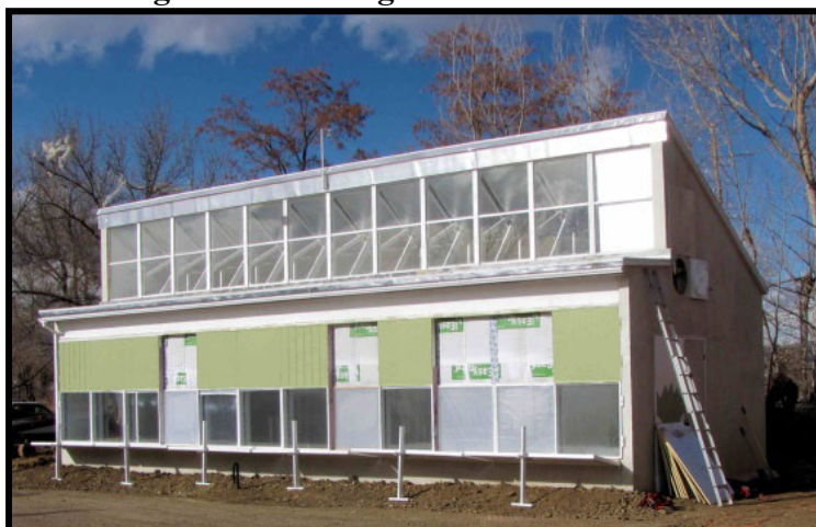
Figure 5. Nearing End of Construction
