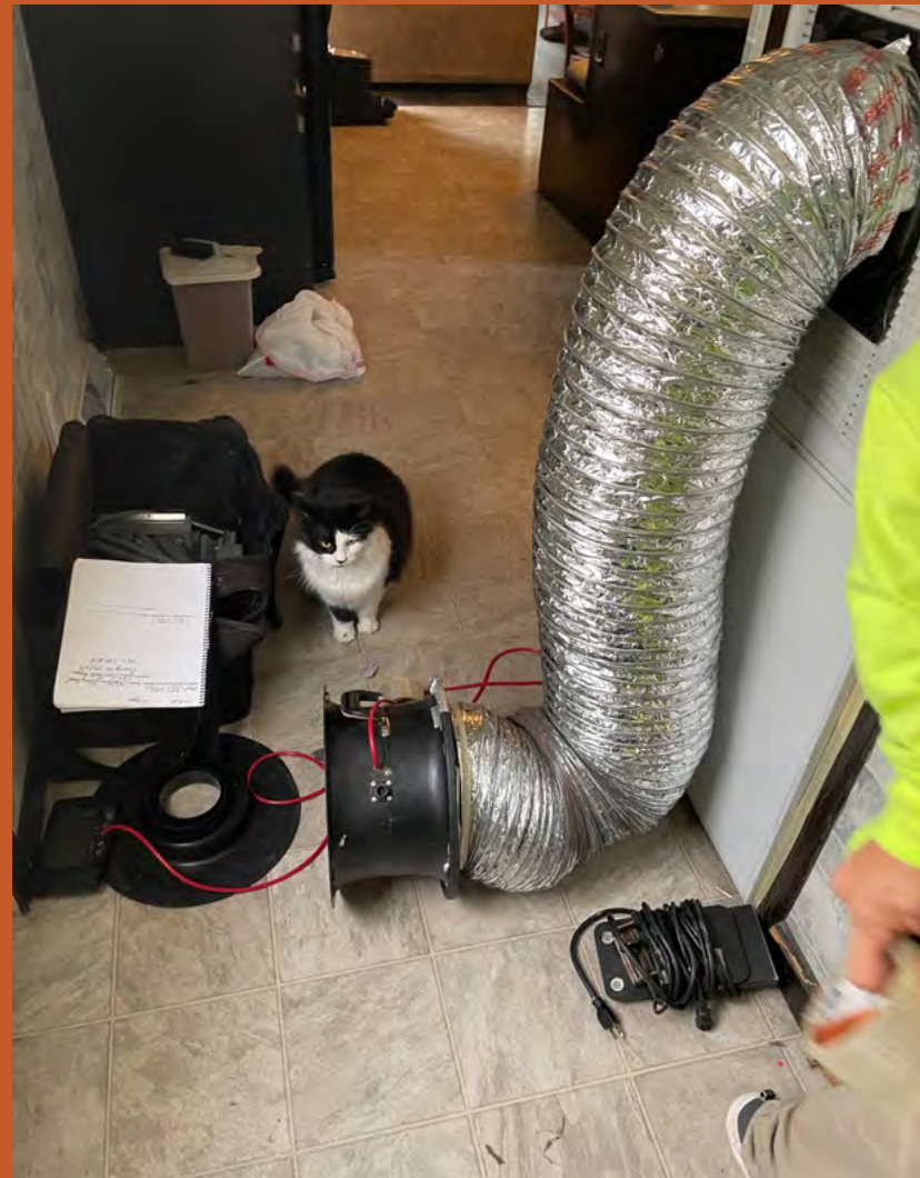
Energy retrofit underway in a manufactured home. Photo credit: Entergy Solutions.
